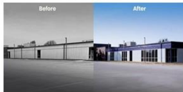
Picture: Before and after pictures of Eisenhower Elementary School. Source: Windows of Opportunity / Windex on YouTube.
